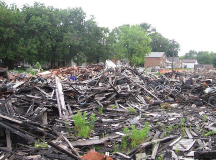
Pictured above: Former Benson Oil Co. site
