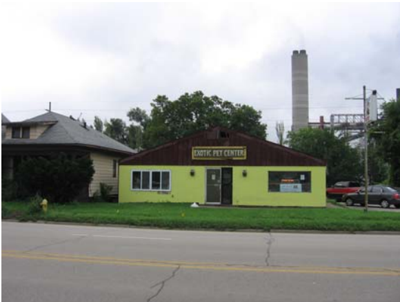
Pictured below: Former commercial/residential sites
